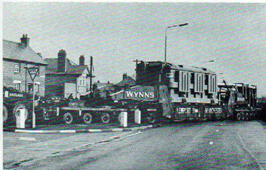
Heavy Load Transporter carrying a 200 ton transformer, operating on a normal road with its skirts raised.
